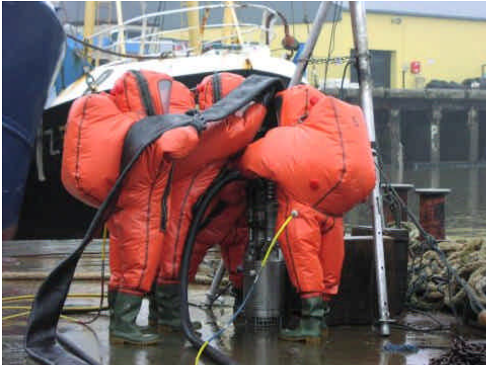
The pump is being connected to the power pack and main hose prior to being introduced into the tank.
