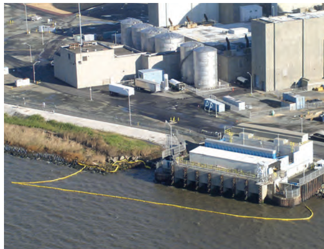
▲ Figure 13: Curtain boom deployed in front of a power station cooling-water intake.
