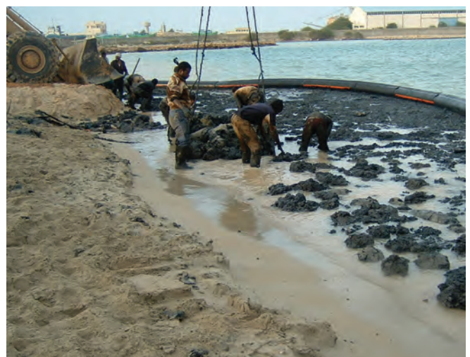
▲ Figure 19: Semi-solid oil held against the shoreline by a section of inflatable boom to facilitate recovery.
