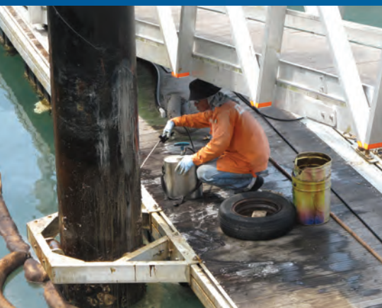
Cleaning pontoon structures at a yacht club, Singapore
